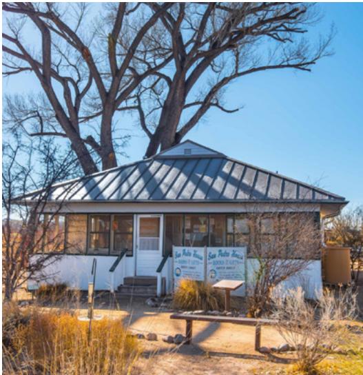
New roof at SPH. Photo by Ron Stewart.
