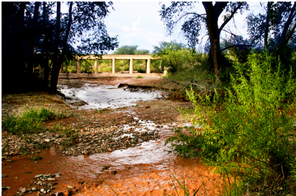
The EP&SW Railroad trestle over the San Pedro River near Lewis Springs. Photo by Robert Luce.
