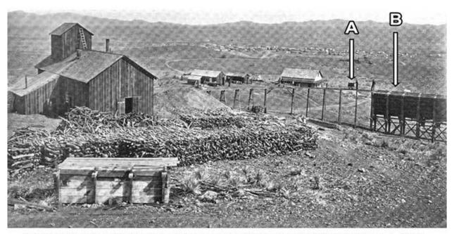
Above. Contention Hoisting Works & Ore Dump, ca. 1880, Tombstone in background. A. Miner returning ore cart to mine. **B**. Ore Bins which when opened allowed ore to fall into wagons positioned beneath. From Tonge, T. 1897., p. 760, 787 abs.
