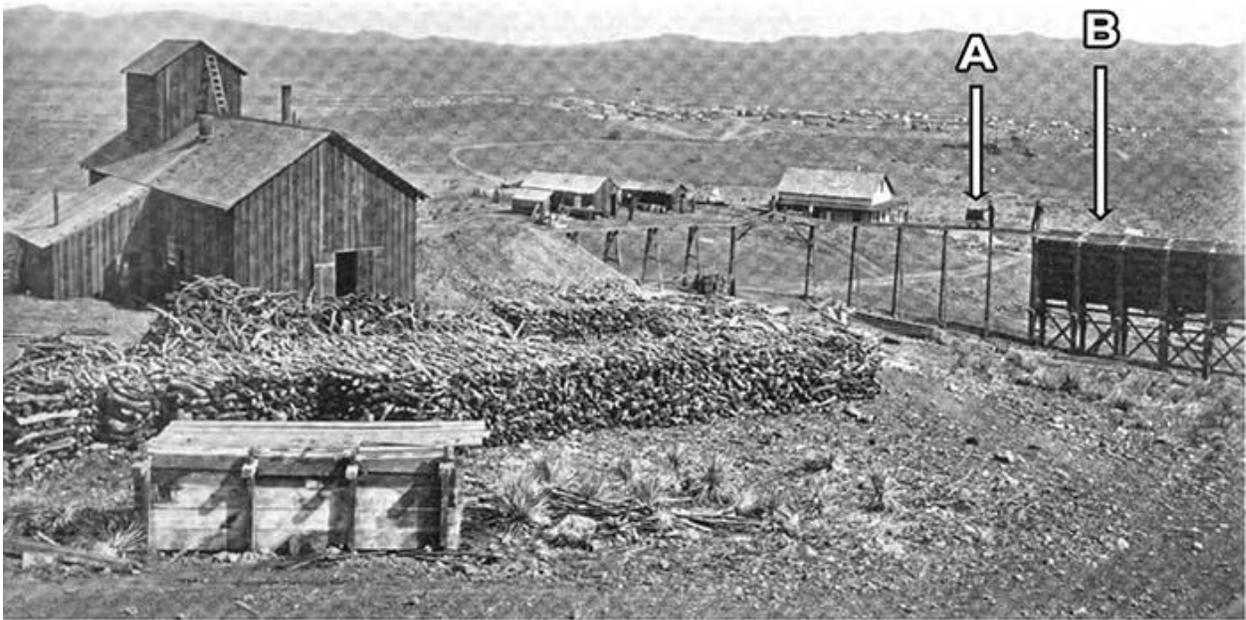
Above. Contention Hoisting Works & Ore Dump, ca. 1880, Tombstone in background. **A.** Miner returning ore cart to mine. **B.** Ore Bins which when opened allowed ore to fall into wagons positioned beneath. From Tonge, T. 1897., p. 760, 787 abs.
